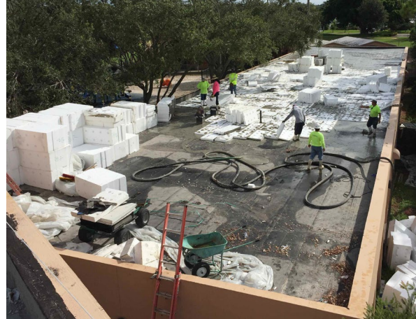
Temporary Membrane Installation
